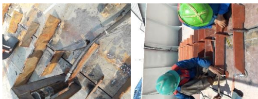
Gambar 8. Fitting Block Metode Stopper Manual.
