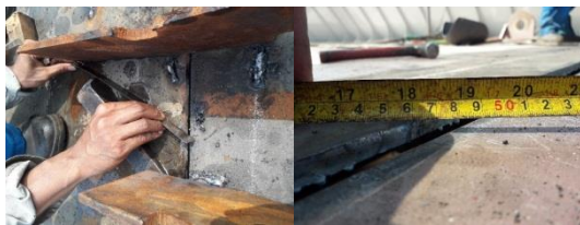
Gambar 7. Adjusting Block Metode Stopper Manual.
