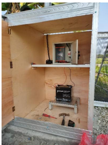
Gambar 7 Rangkaian sistem kelistrikan charging station
