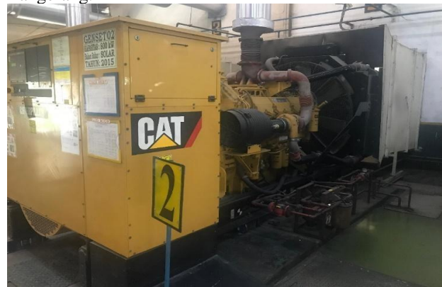
Gambar 2. Genset Caterpillar Type C 32
