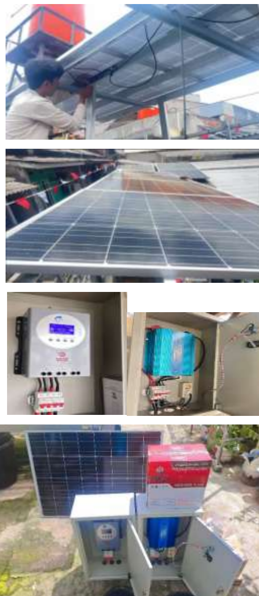
Gambar 3. Proses Pemasangan Panel Surya Instalasi Internet of Things (IoT)
