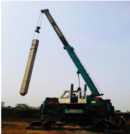
Gambar 3 Lifting pile Sumber: Arif Rahman Hakim, 2018
