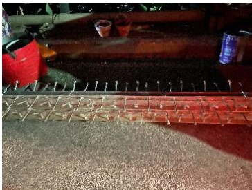
Gambar 2. Sambungan Tipe Strip Seal
